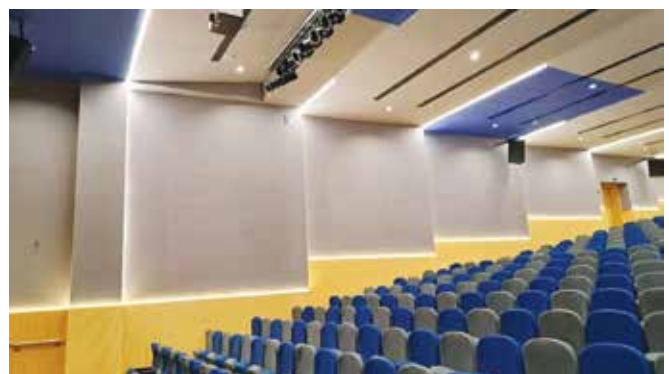
Educational auditorium at Reva Institute of Technology & Management [RITM] Bengaluru Acoustical panelling with a combination of Strand Slim and Slats Surco backed by SynthPF Dissimilar materials create impedance mismatch that results in broadband sound absorption
