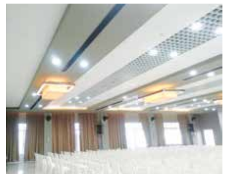
Multipurpose hall for Lourdes Public School & Junior College by Lourdes Educational Trust at Kottayam [Kerala].
