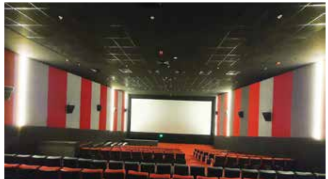
Y Screens, Jangareddigudem [Andhra Pradesh] Ceiling with Subtlex Ebony on Skelet Ebony T-grid Panelling with Tufbloc HDFR, SynthPF and Strand backer.
